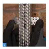
• Bend back protruding bracket legs to sit clear of the channel face.
