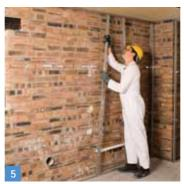
• Cut Gypframe GL1 Lining Channels to size and round-off ends with tin snips for an easier fit.
