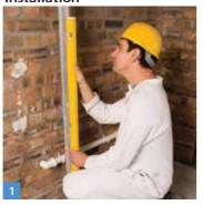
• Use a straight edge (e.g. Gypframe GL1 Lining Channel) to determine the maximum undulation in the wall or service protrusion. This will determine the cavity depth.
