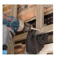
Position short lengths of Gypframe GL1 Lining Channel above the opening for additional support and to maintain appropriate support centres, and fix using two Gyproc Wafer Head Drywall Screws
