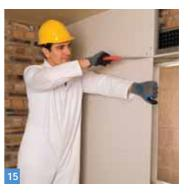
• Where door openings occur in the run of lining, cut board around the opening to avoid a joint directly in line with door jambs.
