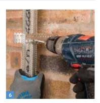
• Bend bracket legs forward and fix each leg to the channel using a Gyproc Wafer Head Drywall Screw. Insert screw through the hole in the bracket nearest to the back of the channel (see Junction detail – 18).
