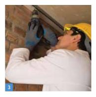
• Fix Gypframe GL8 Track to perimeters, with the longer leg towards the lining, at 600mm centres using appropriate fixings (see Base detail 20).
