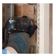
• Fix Gyproc edge bead to the perimeter of the window frame to provide edge protection to the reveal and soffit linings.
